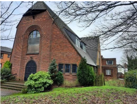
Figure 1. Primary elevation as viewed from St Columba's Close
